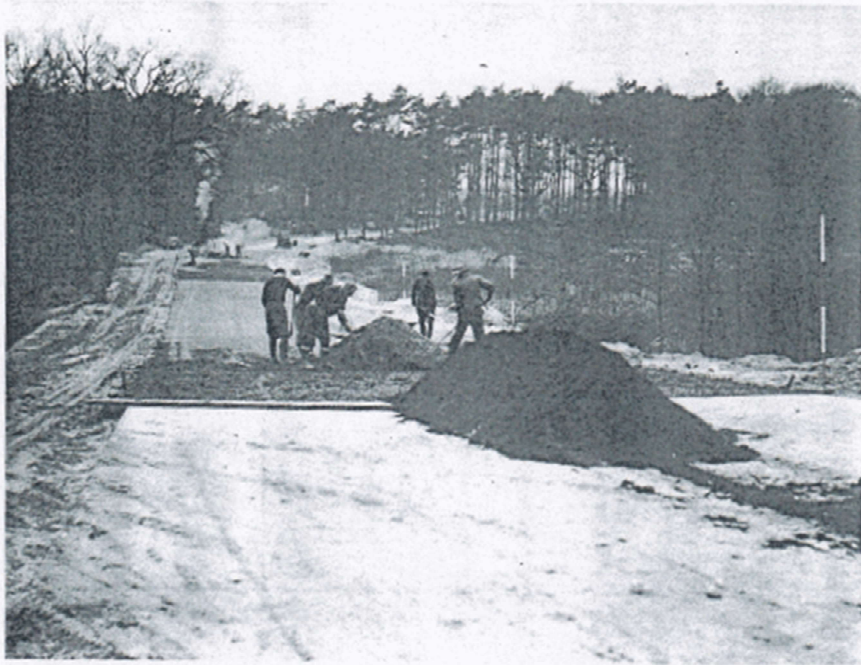
Photo 14.—Laying the first roads.
