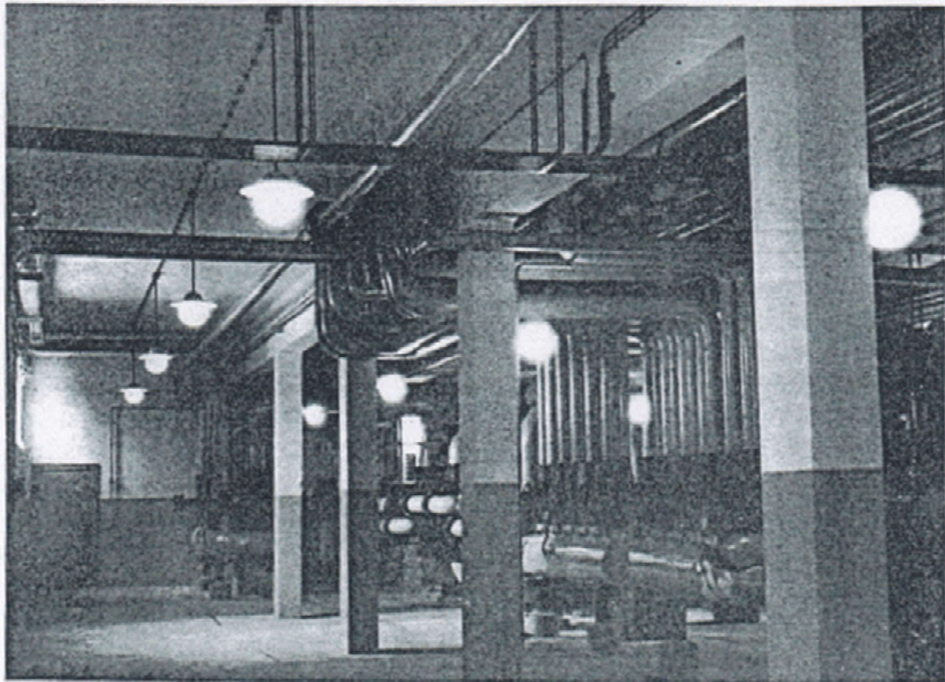
Photo 9.—Calorifier station.
